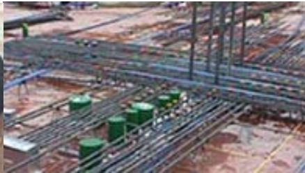
DECON® Studrails can simply be placed alongside openings to create a continuous stress path to the column.
