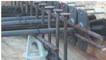
DECON® Studrails greatly reduce reinforcement congestion in thin PT slabs
