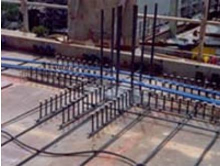
Easy location of DECON® Studrails to flat slab formwork at column locations. They enable drop panels, beams and column capitals to be removed from the design.
