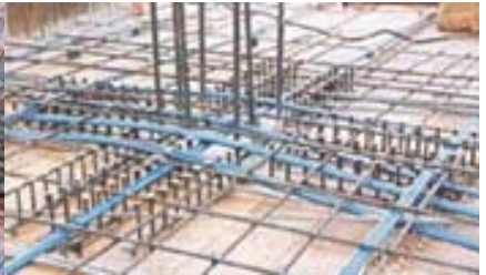
Typical finished layout of DECON® Studrails, rebar, and PT tendons at column/slab interface
