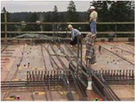
Easy location of DECON® Studrails to flat slab formwork at column locations. They enable drop panels, beams and column capitals to be removed from the design.
